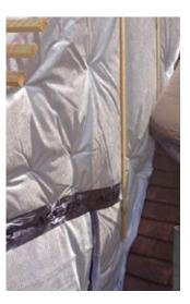
**5** Fix horizontal tiling battens to size and gauge in accordance with tile manufacturers requirements, usually 38 x 25mm minimum.
