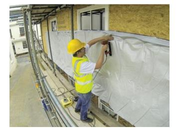
**3** Fix next layer to support, overlapping the product by 50 - 100mm. Ensure all joints are taped using **ACTIS Multidhesif**.
