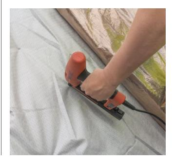
If installed directly onto rafters it is recommended that BOOST<sup>\*</sup> HYBRID is pulled taut and counter battens (38 x 25mm minimum) are fixed in line with rafters before tile battens, to guarantee a clear drainage path for rainwater.
