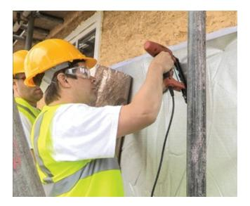
2 Staple to the structure using galvanised staples (minimum 14mm) every 50mm keeping insulation as taut as possible.
